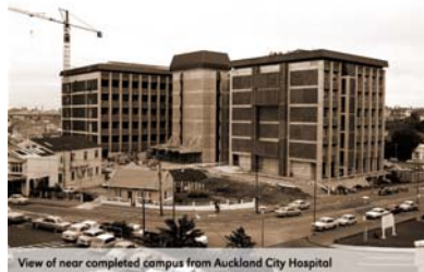
View of near completed campus from Auckland City Hospital
