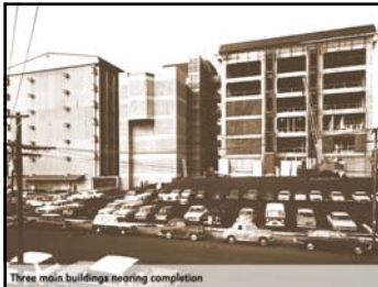
Three main buildings nearing completion
